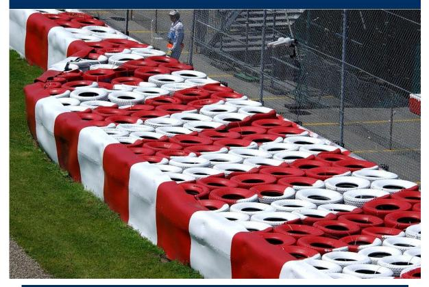
The use of tyre barriers on motor racing circuits is an effective means of absorbing the energy of a vehicle in the event of a collision, but only when constructed according to the latest best practice guidance provided by the FIA and its Circuits Commission.
